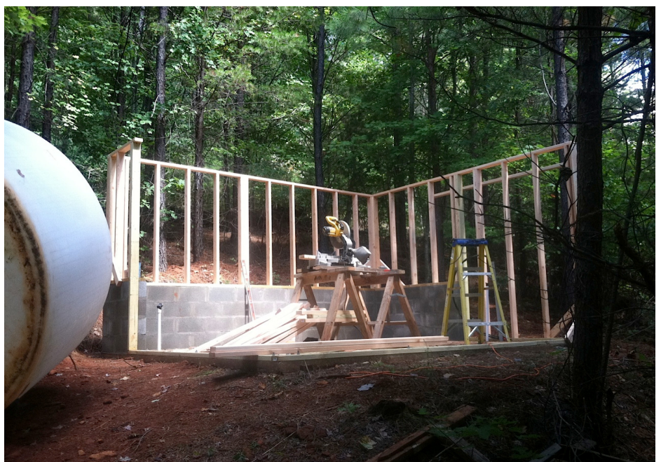
Pump House under construction (Home for the 1550 gallon water reservoir)
