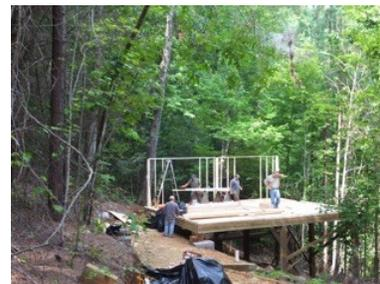
*The framing crew at work after the concrete had been poured and support posts erected in August 2016.*
