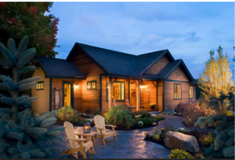
Shepherd's Cottage is well underway!
